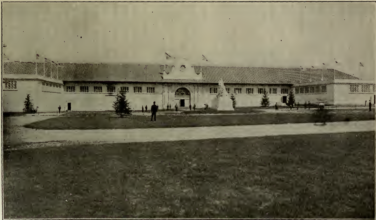
MACHINERY, ELECTRICITY AND TRANSPORTATION BUILDING 100 x 500 feet, with wings on either end 100 x 100 feet each.
